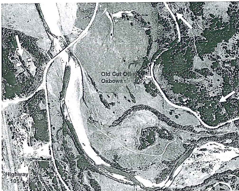
Figure 12-2. Aerial photo of Pistol River showing confinement by a levee. The levee separates the active channel from adjacent farm and industrial gravel operation to the west (left). The levees also cut off the river from oxbows and meanders on the east bank (right), which would have formerly created ideal coho salmon rearing areas. Yellow arrows highlight pockets of residential development.
